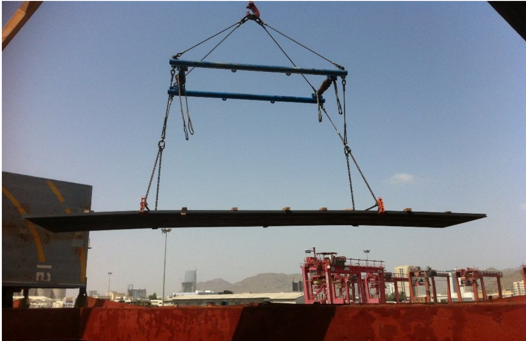
1 st Batch of Steel Plates
