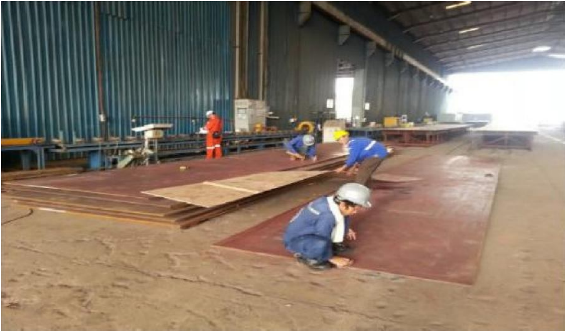
Plates marking of the tank plates are on-going at Batam Workshop
