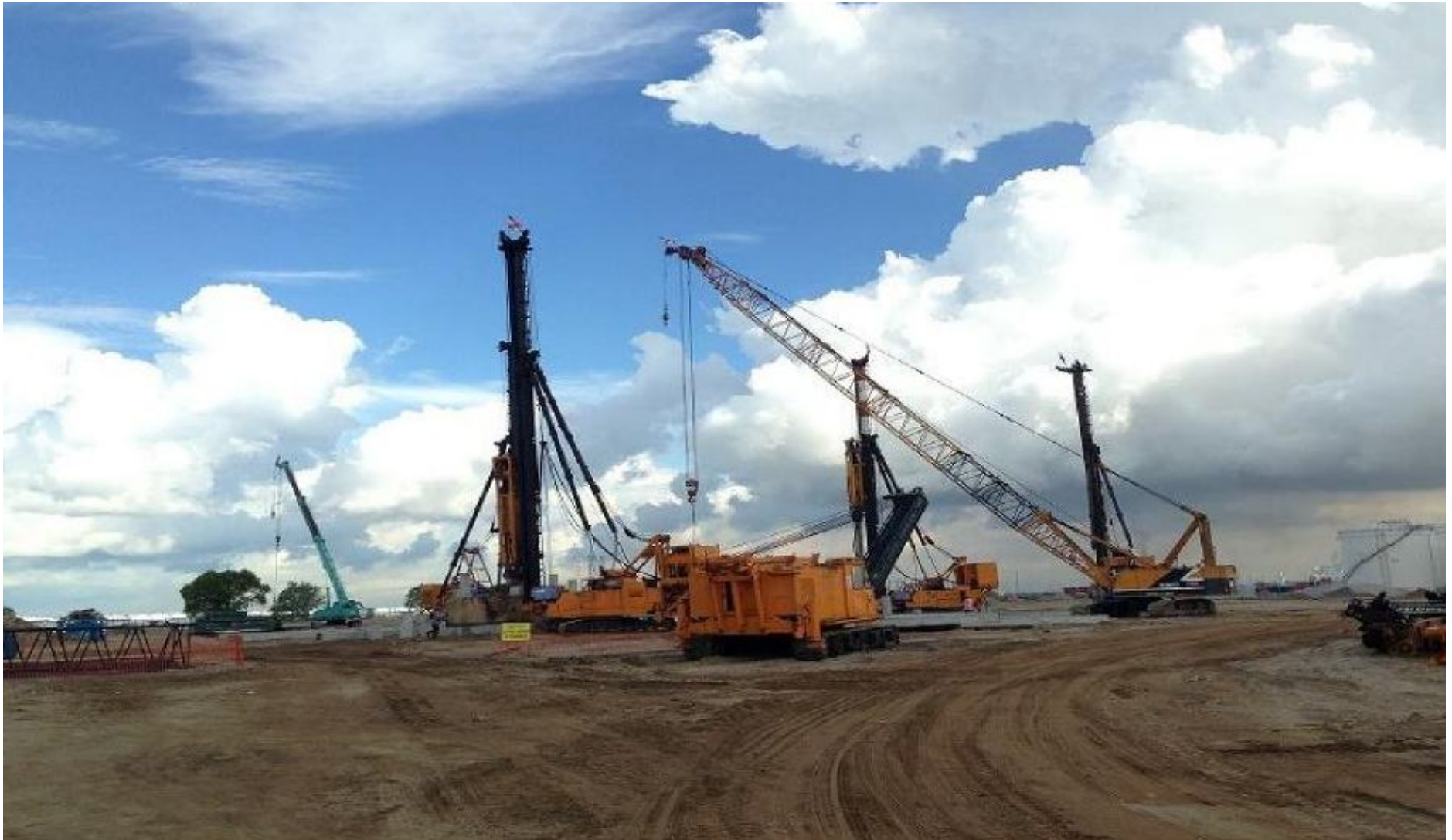
Piling works activities at Pit-46
