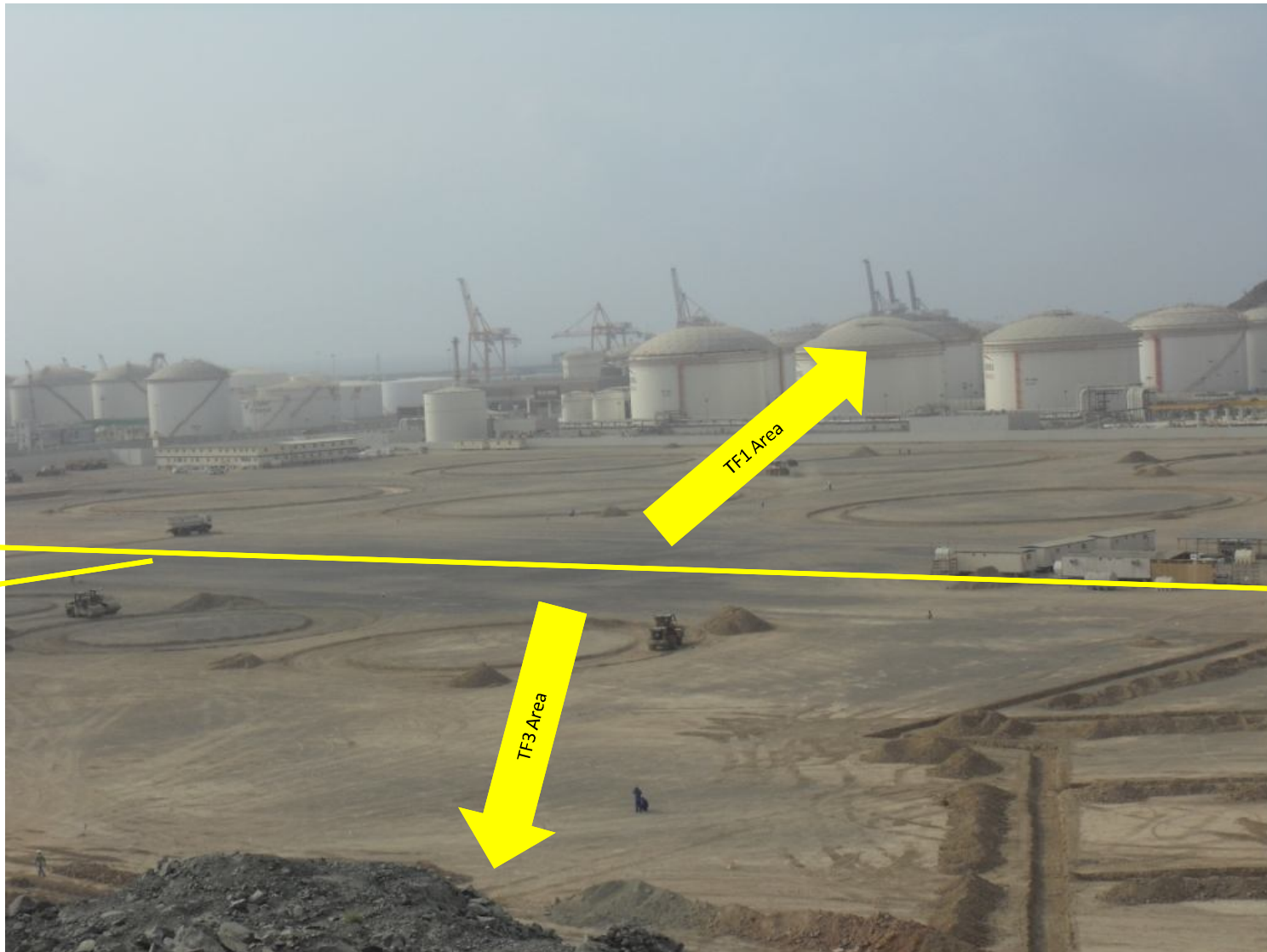
Tank foundation and bundwall works in progress
