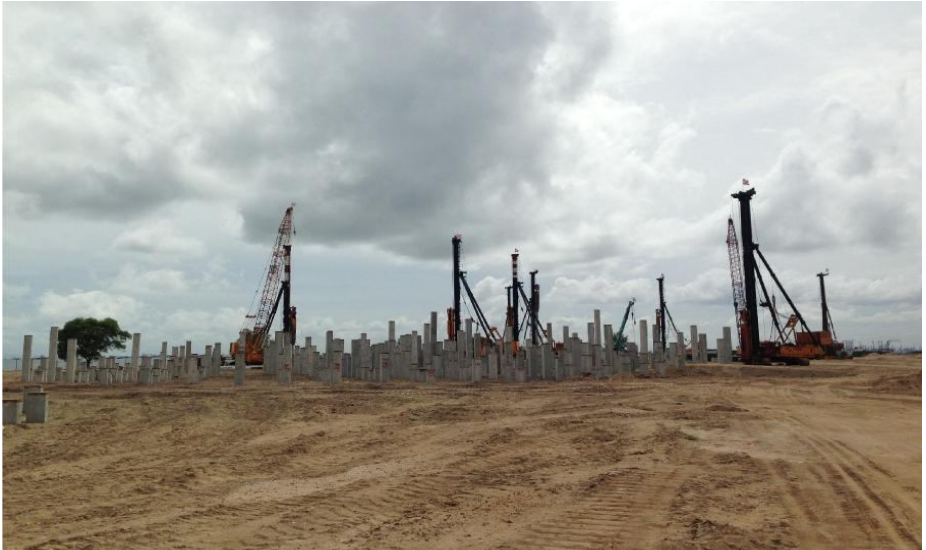
Piling works on-going
