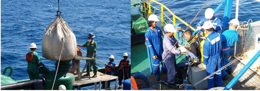
Loading of cement into cutting pot
