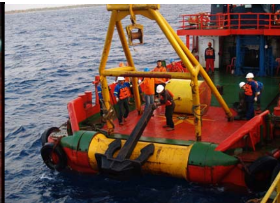
Anchoring Work
